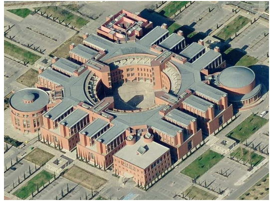
Fig. 1. Building with a complex layout: The Engineering School of the University of Alcalá-de-Henares (UAH) in Spain.
